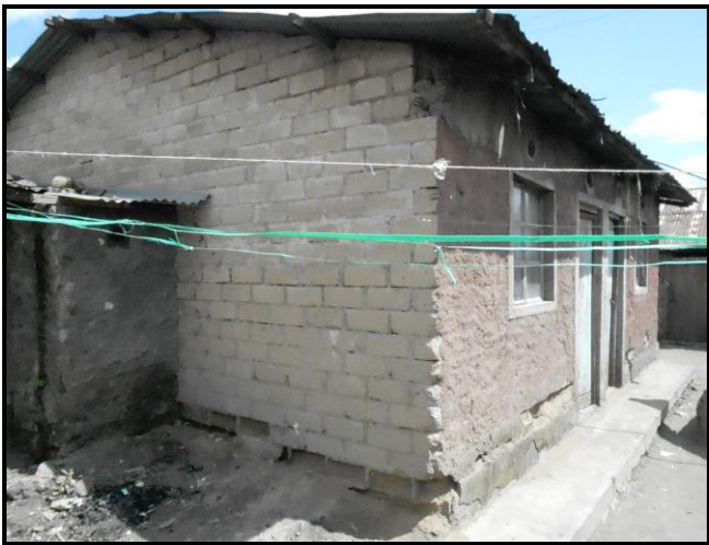
Plate 4.5.7: Status of a Project House at the Time of the Study
