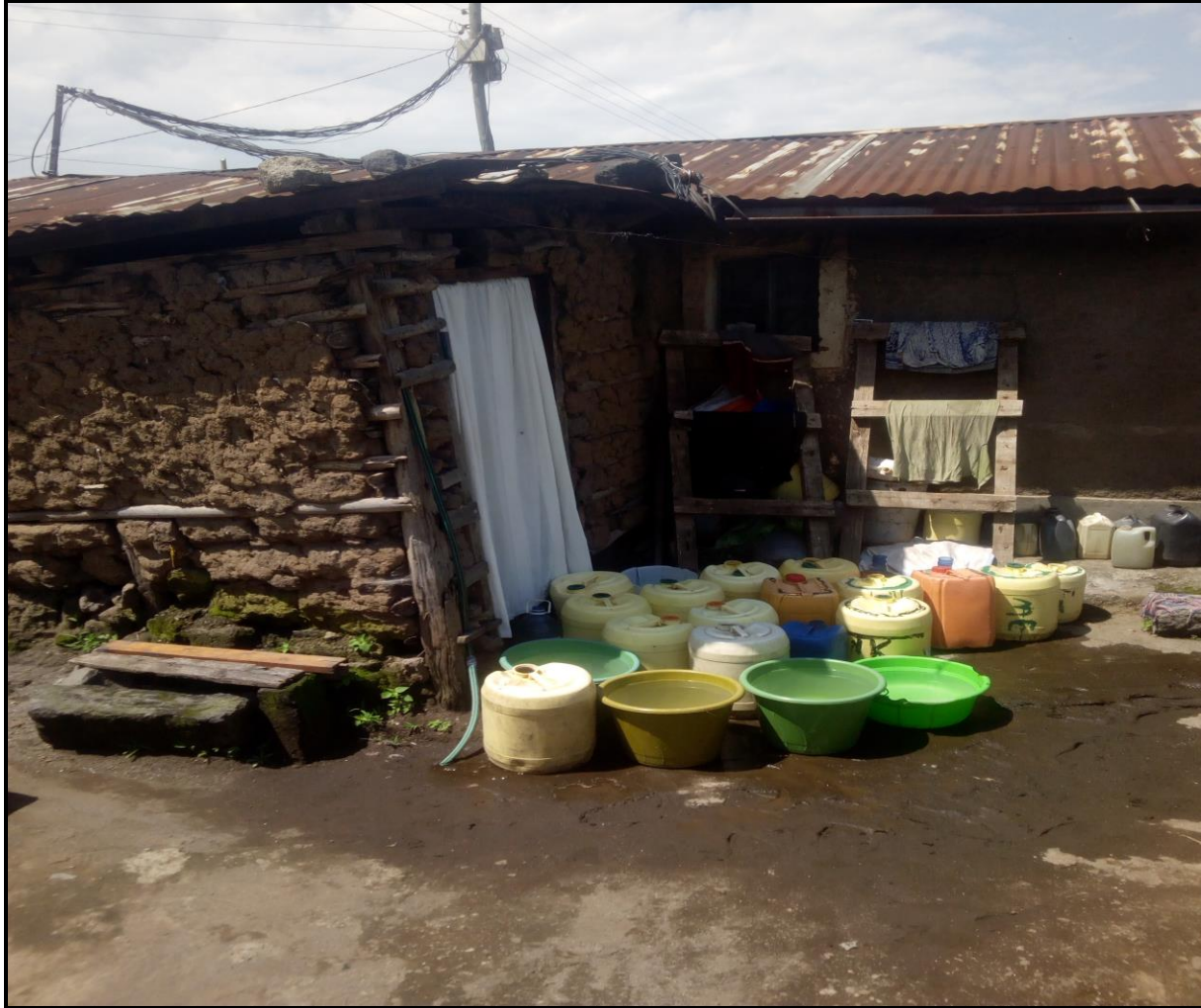
Plate 4.7.2: Illegal Water Connections in Kwa Rhonda Project Site
