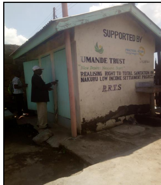
Plate 4.5.4: Ventilated Improved Toilets in Kwa Rhonda Project Site
