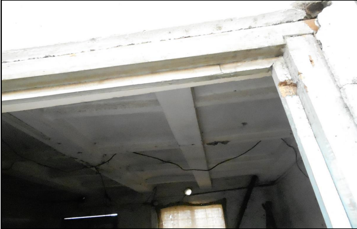
Plate 4.7.12: Lattice Precast Flooring System in Lake View Project Site
