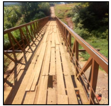
Status of the bridge 15 years
