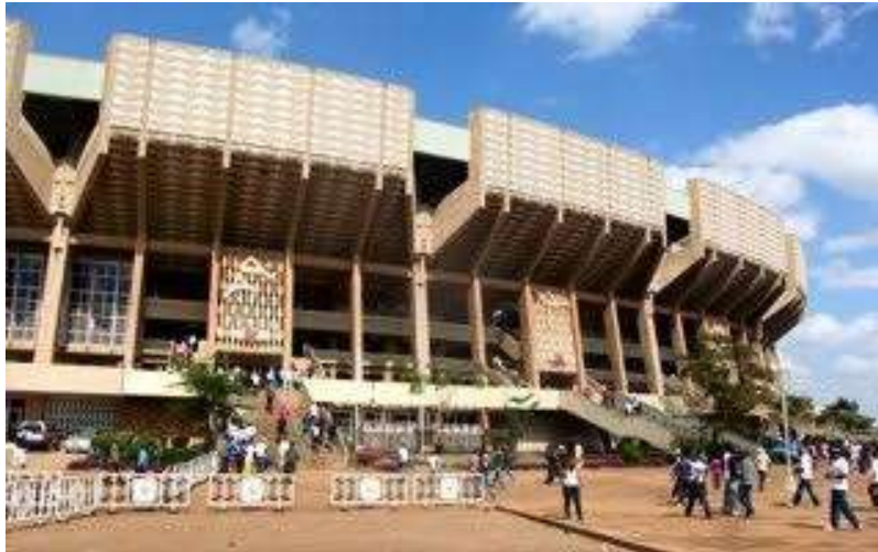
Fig. 5.3 The face of main entrance to Moi International Sports Centre Kasarani before commercialisation of sports in Kenya
