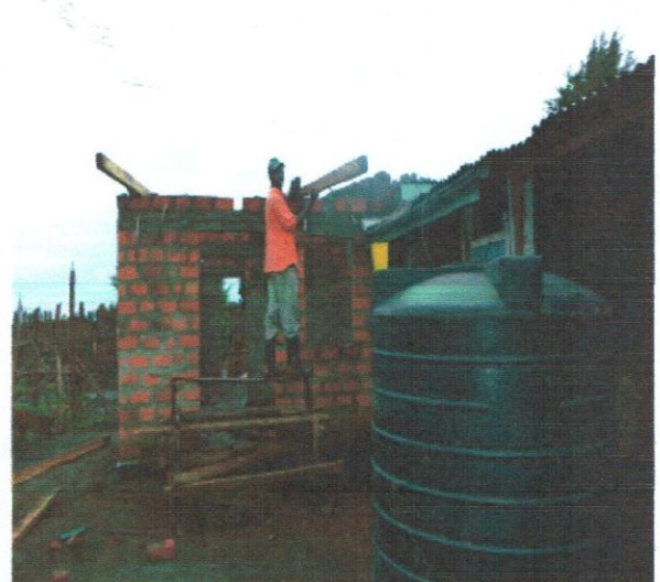
Tanks for water harvesting in Amalo Location.
