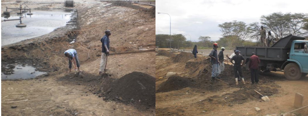
Plate 2: Unprotected workers removing silt and solid waste from one of the waste water treatment ponds in Nakuru County.
