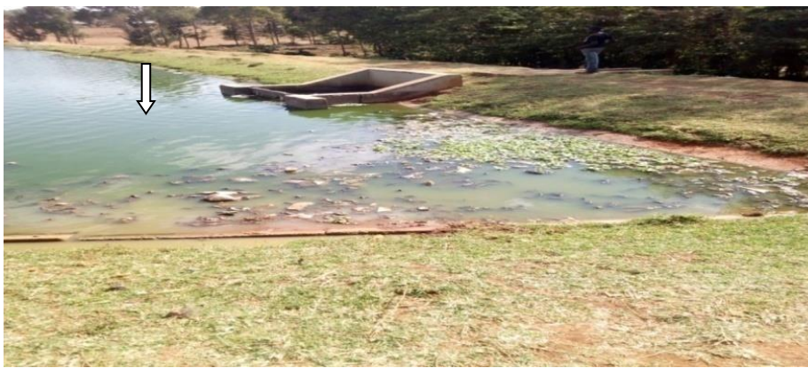
Plate 4.9: Algae Bloom in the Last Maturation Pond of Huruma Treatment Plant an Indicator of High Nutrients in Treated Effluent Water Discharged into Sosiani River.
