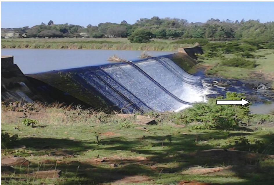
Plate 4.1: Two River Dam in Kaptagat Forest the Source of Sosiani River Fenced and Protected from Human and Livestock Encroachment
