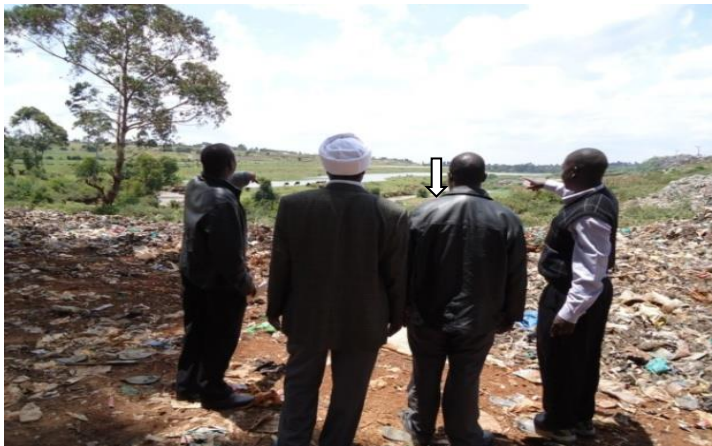
Plate 4.8: NEMA Officials Inspect Water Pollution along Sosiani River between Huruma Dumpsite and Huruma Effluent Treatment Plant.
