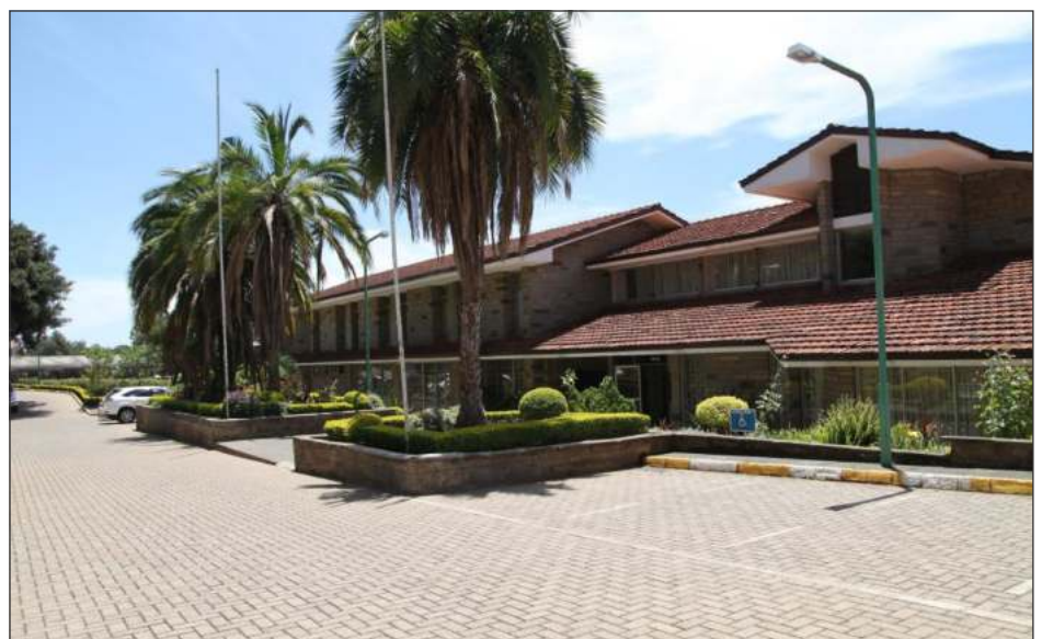
The ARC Hotel at the Njoro Campus, one of the units under EUICO
